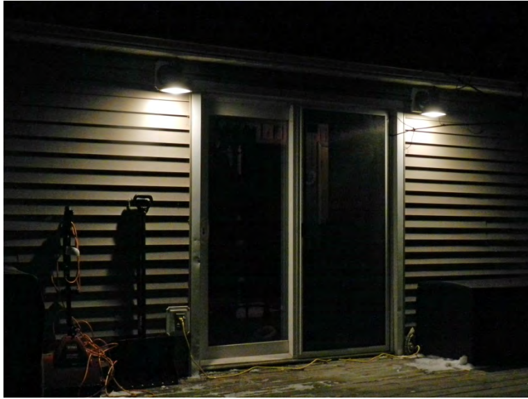
Patio Lights at Night After Replacement with Fully Shielded Lights
